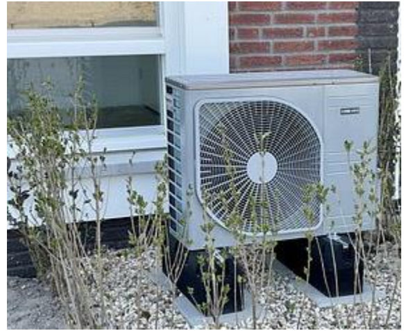
The outdoor unit of a heat pump system.
